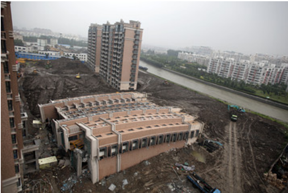
Bloomberg News The collapsed building, which has since been demolished
