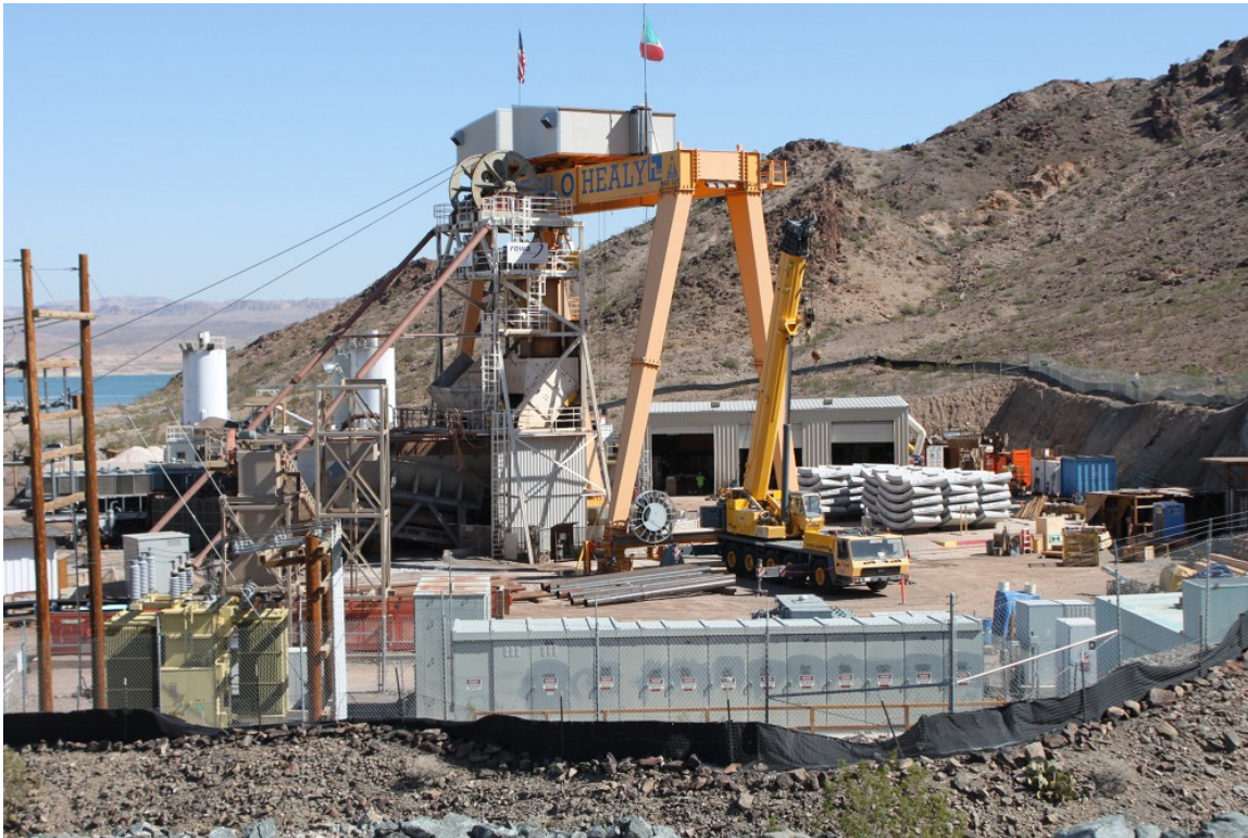
Segments await gantry lowering into 18m deep shaft at the launch site
