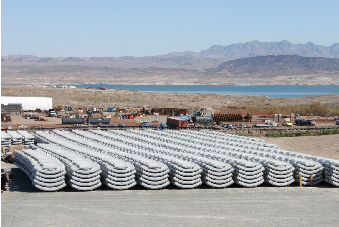
All that remains of an initial 2,500 x 6 segment stacks
