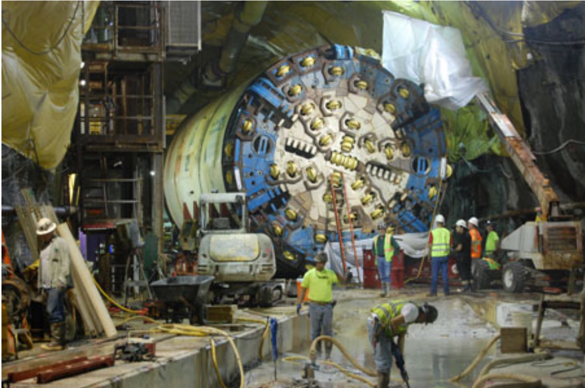
Lake Mead TBM readied for its drive under the lake
