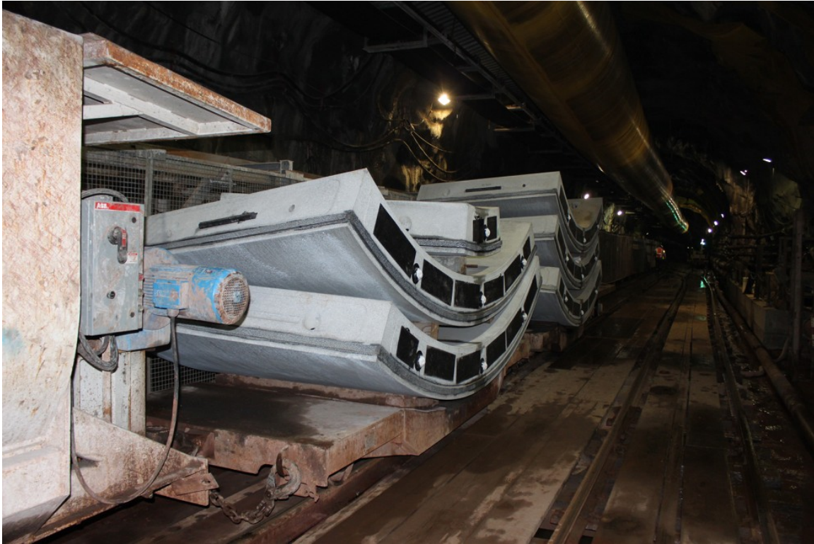
Six tunnel segments, which form a ring and 1.8m of progress, on a flat car for a ride to the tunnel heading
